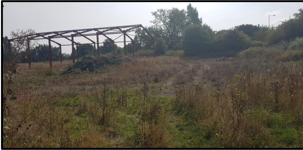
Figure 2: Frame of former light industrial unit
