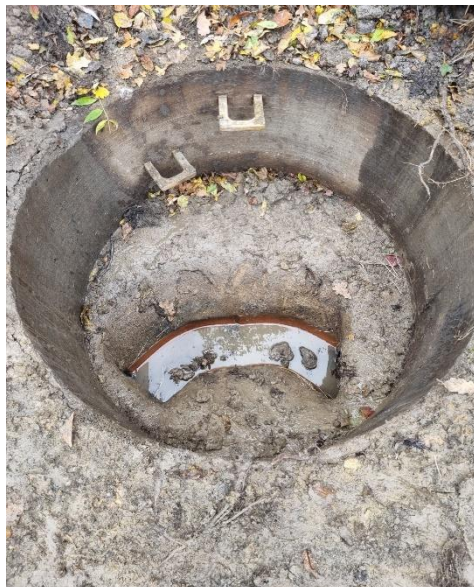
Figure 13 Chamber 2 on the Site Boundary
