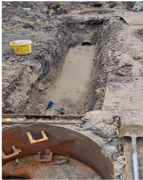
Figure 15 Drainage Run Between Chamber 2 and Chamber 3
