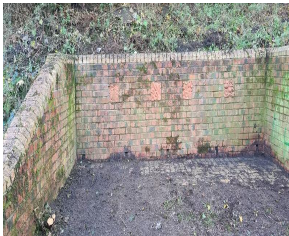
Figure 17 Brick Enclosure on West side of Trans Pennine Trail
