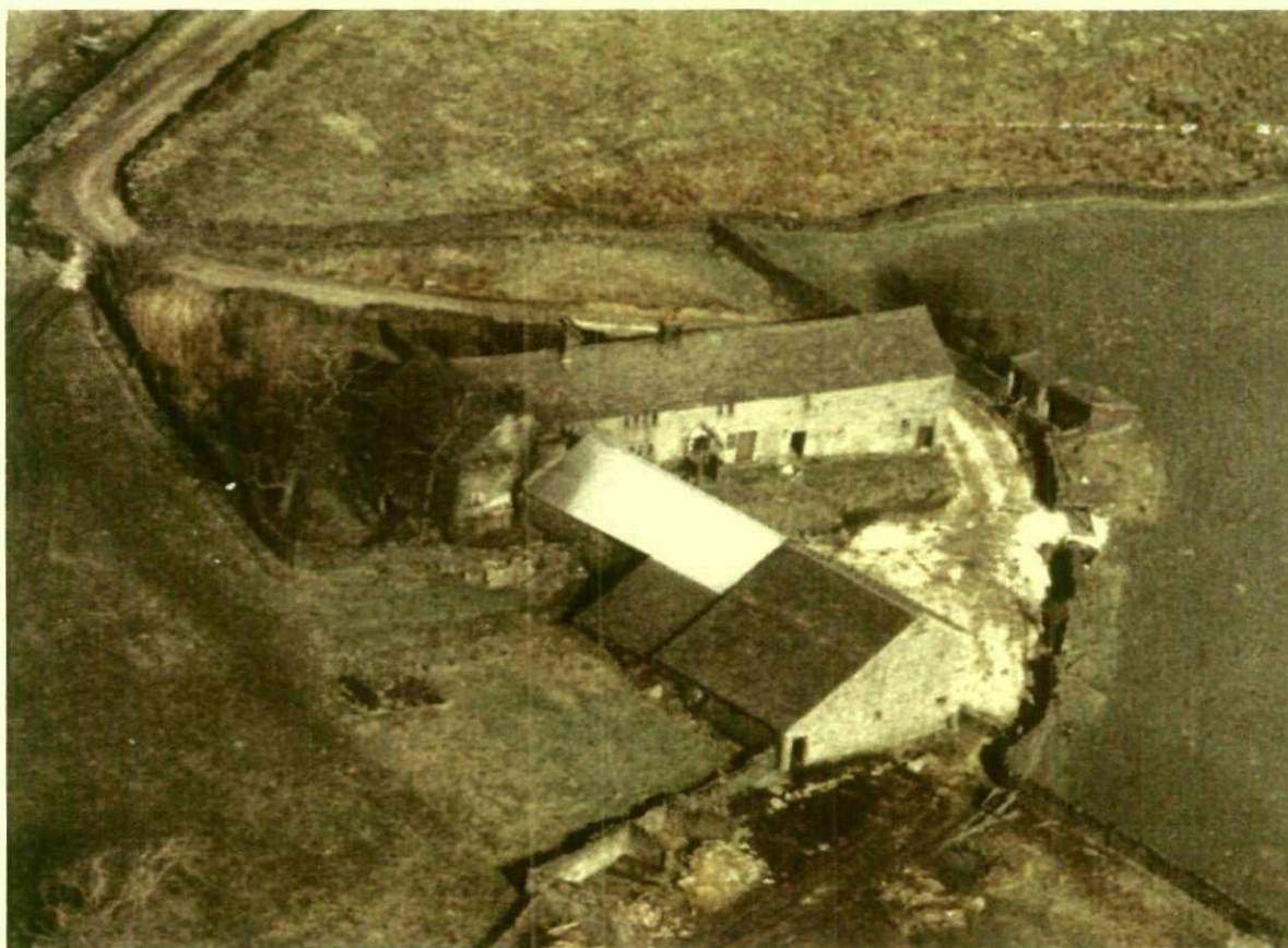
Aerial view of farmstead showing original lean-to.
