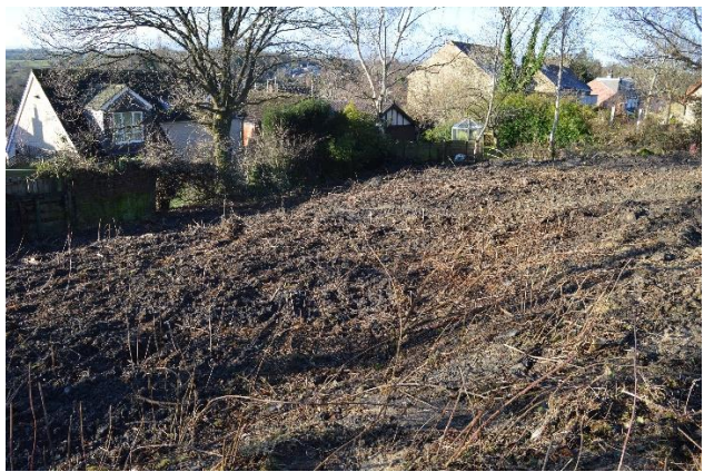
Figure 13: The cleared site, January 2025
