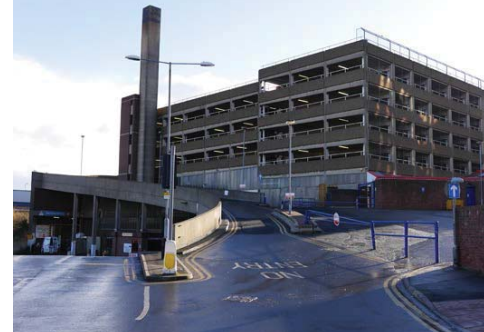
Multi-storey car park viewed from jumble lane crossing
