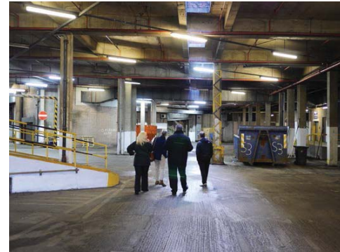
Metropolitan Centre - View of basement
