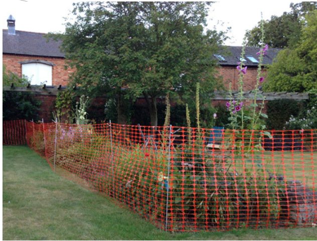
Plastic mesh tree protection fencing
