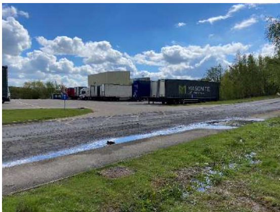
Photo 7: View looking east towards lorry park – note water issuing at surface on western plot
