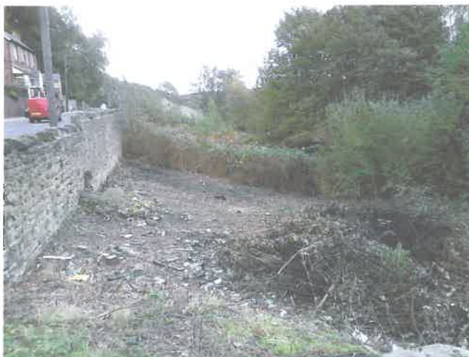
Photograph 1 General site view
