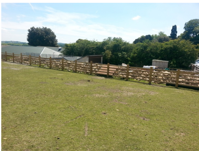
General Building scale of Farm Buildings below the existing tree line
