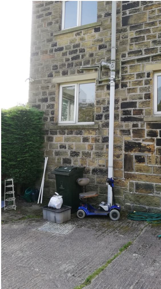
View of the north elevation
