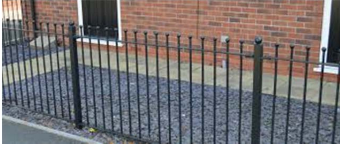
Typical appearance of fencing
