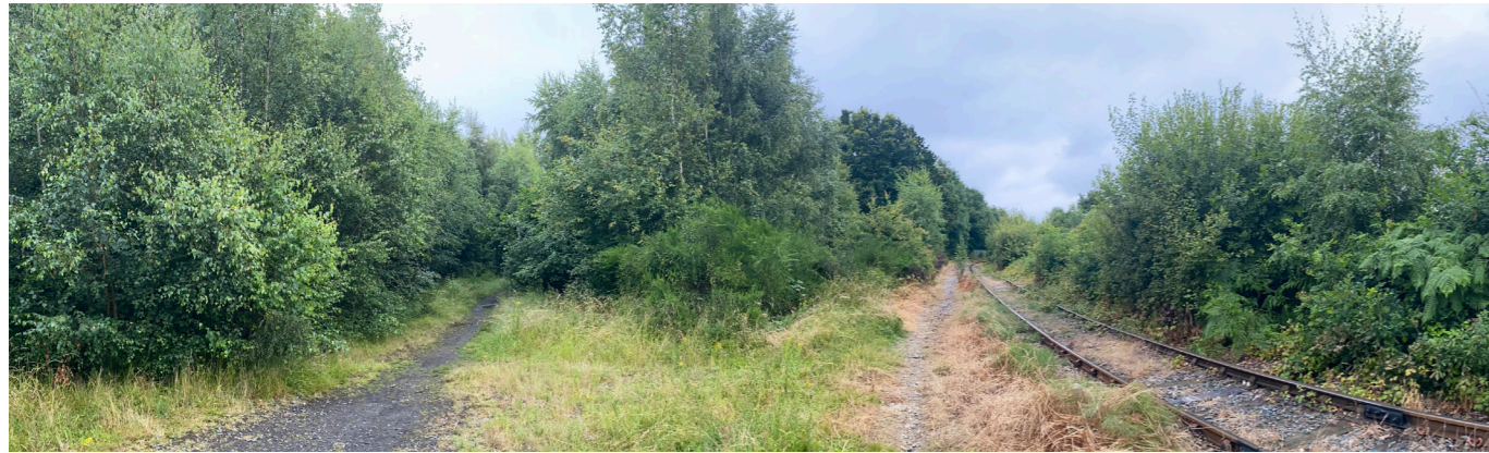
View from permissive path and rail line
