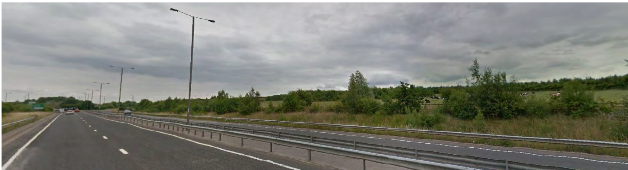
Existing street View looking East at Phase 2 Land
