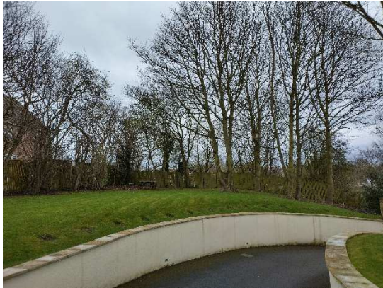
Photo 1: T1 to G8 from west
