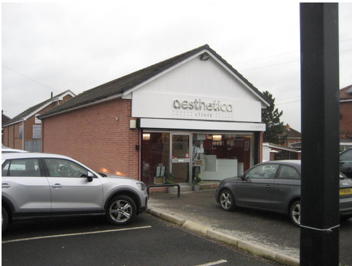
A view of the existing building.
