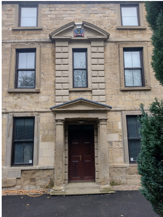
Fig 2: South Porch and Portico
