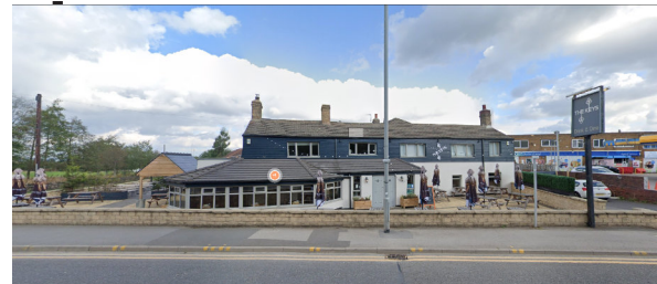
Render with painted timber cladding
