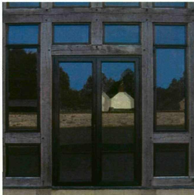
Steel casement window
