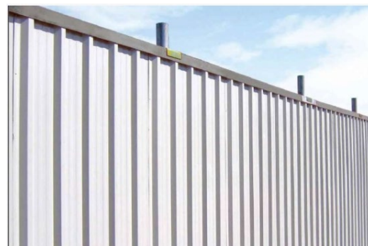
Example above showing tree protection fencing by the use Heras Steel Boarding. https://www.heras-mobile.co.uk/fencing/steelboard
