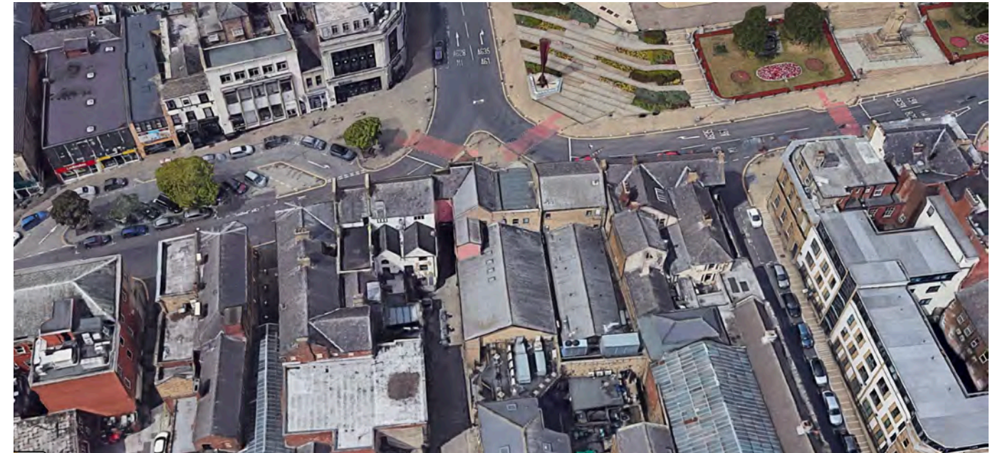
Site Aerial Looking West
