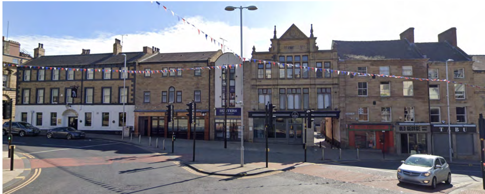
Existing Building Frontage From Approach On Shambles Street
