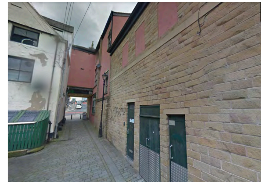
Existing Rear Access From George Yard
