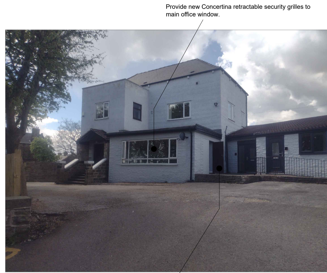
Photo 1: Form new wheelchair accessible entrance to side door. Widen opening as required and provide new PVC doorset to comply with AD Part M. Modify ramp and landing / handrail balustrade (extend as required).
