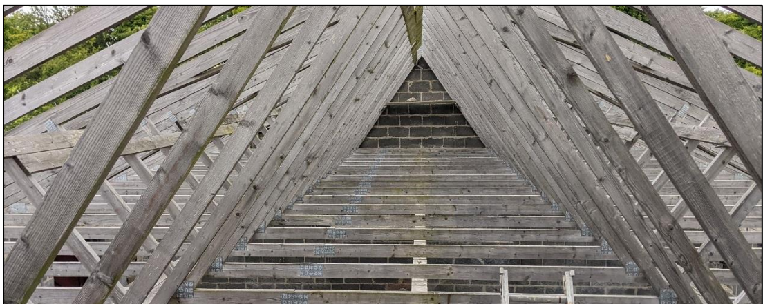
Plate 4. Pre-formed trusses in roof structure of former stables
