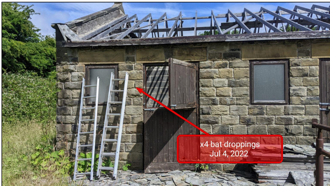
Plate 4. Pre-formed trusses in roof structure of former stables
