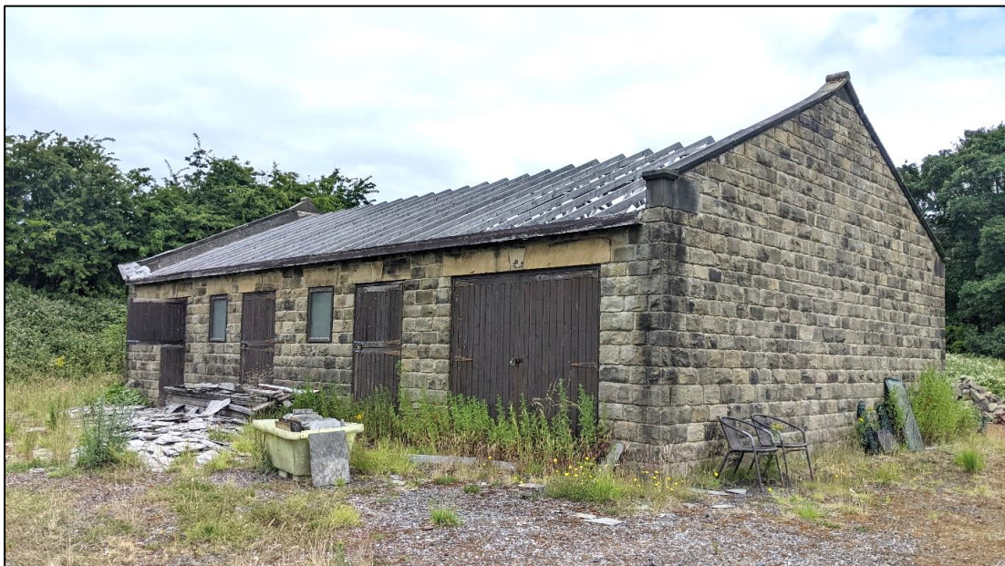
Plate 1. Southeast corner of former stables
