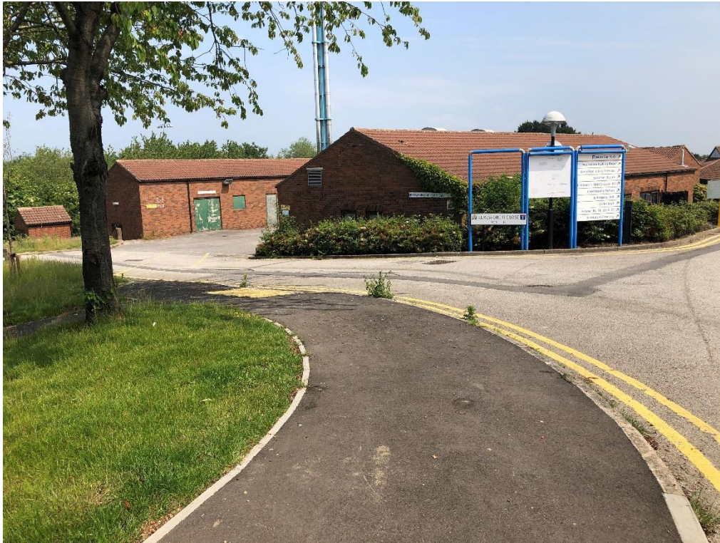
Photograph 1: View of the Keresforth Centre (facing north-east)
