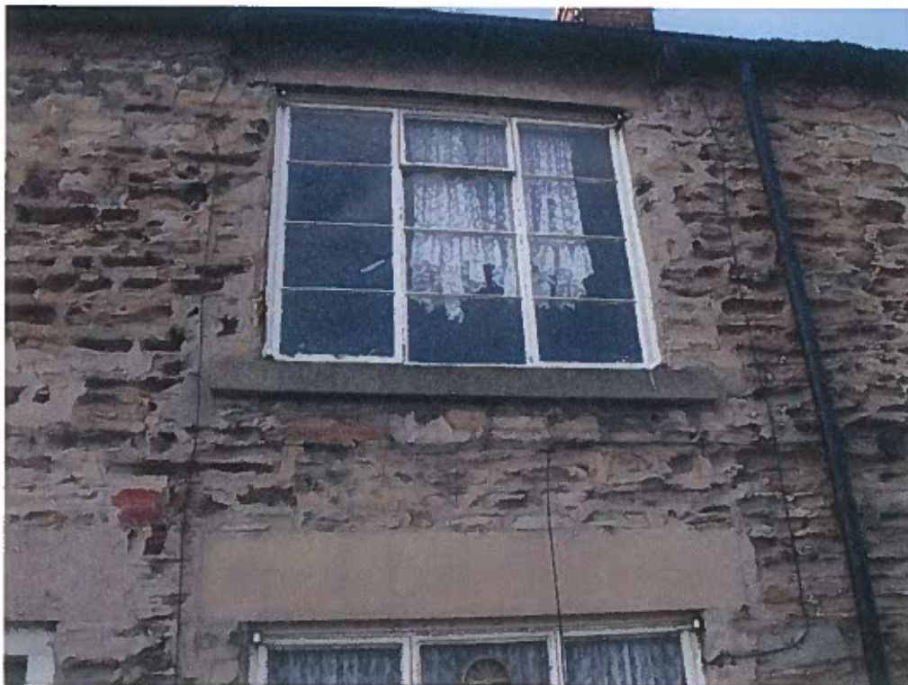
Photo 5 Front Elevation 74 Wath Road
