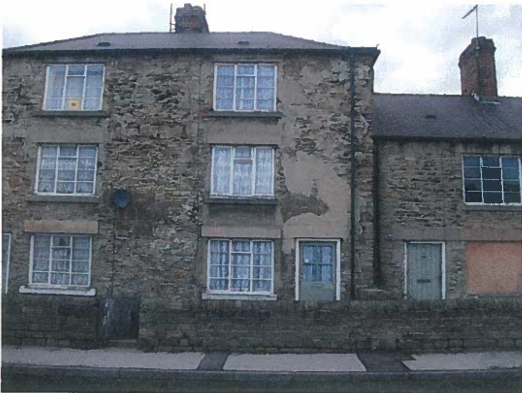
Photo 1-Front Elevation 70+72 Wath Road
