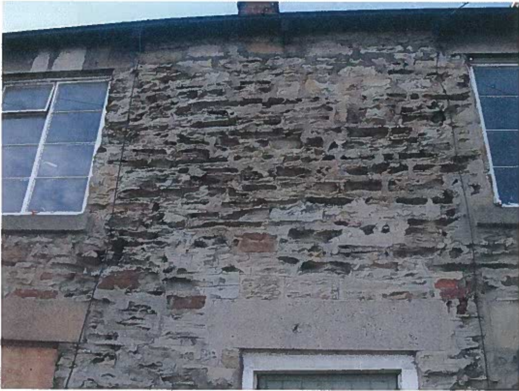
Photo 2 Front Elevation of 72 Wath Road at First Floor level
