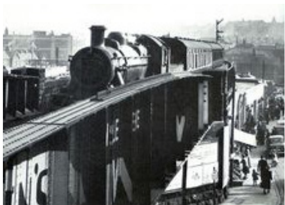
A train crossing over the former bridge over the corner of Regent Street and Eldon Street overhead.
