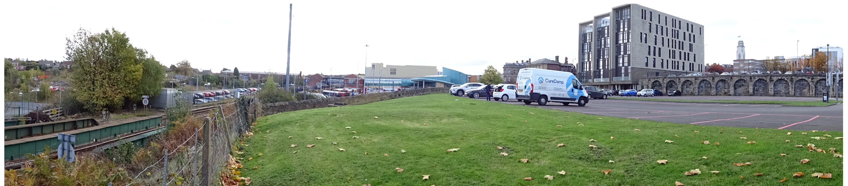
Figure 7.2: Panoramic view of part of the Lower Courthouse, looking south west
