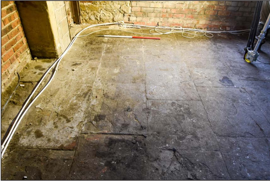
Image No. 23 Film No. Darley Cliffe Hall_021 Direction: E Description: Stone flagged floor in the north east quadrant of the room
