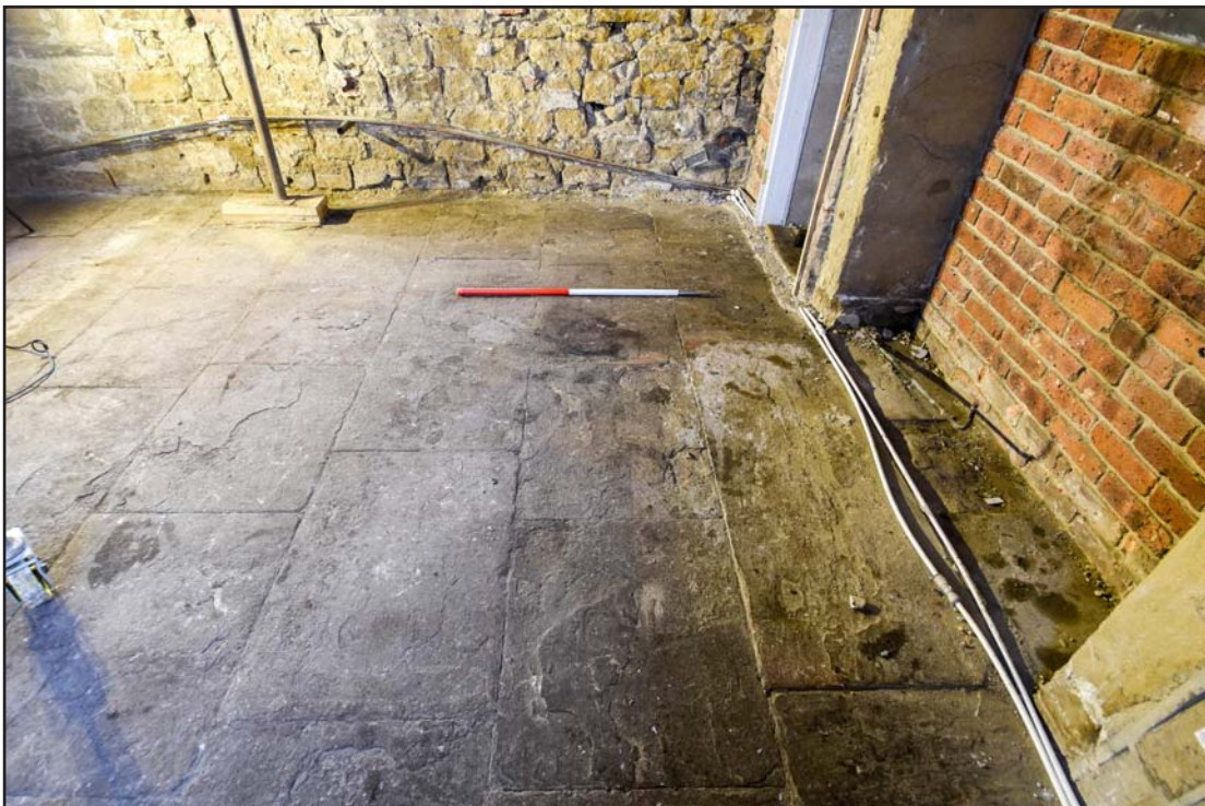
Image No. 24 Film No. Darley Cliffe Hall_017 Direction: W Description: Stone flagged floor in the north west quadrant of the room
