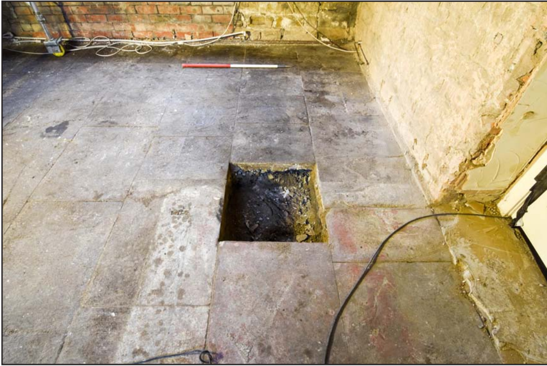
Image No. 21 Film No. Darley Cliffe Hall_018 Direction: NE Description: Stone flagged floor in the south east quadrant of the room
