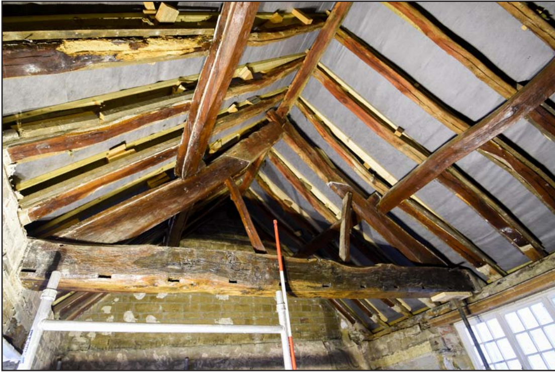
Image No. 13 Film No. Darley Cliffe Hall_016 Direction: SW Description: North face of the truss
