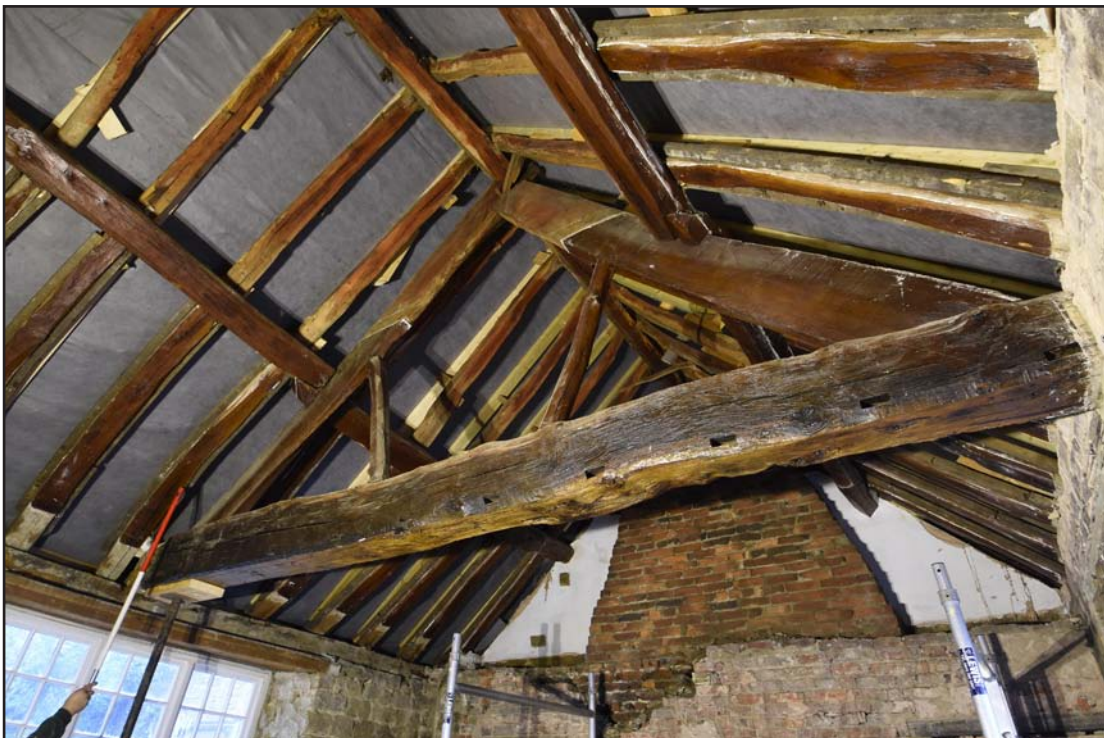
Image No. 14 Film No. Darley Cliffe Hall_020 Direction: NW Description: South face of the roof truss
