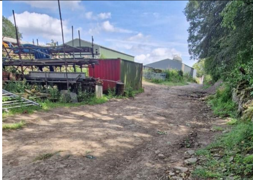
View looking East along access track towards Gunthwaite Barn
