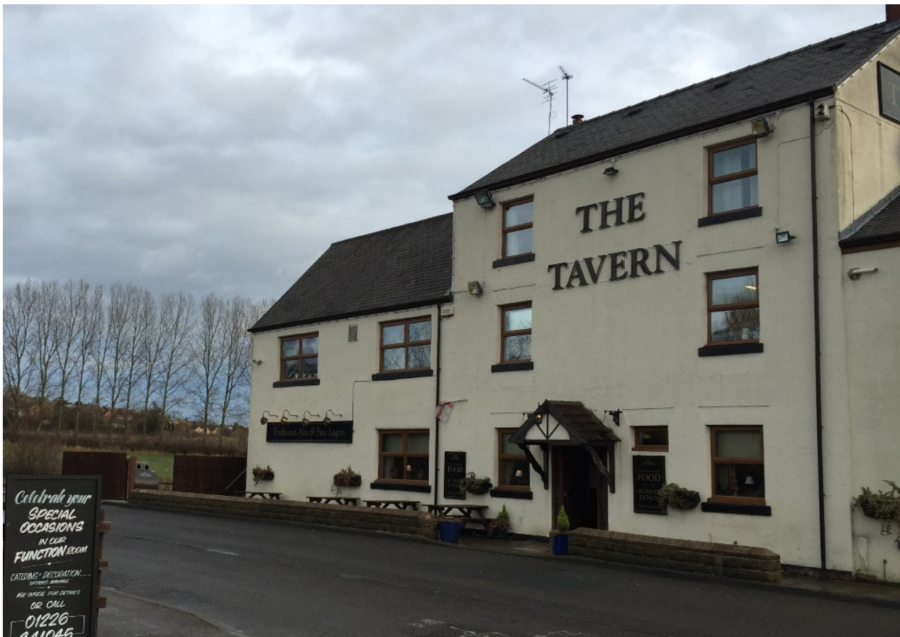
View to the front left hand side elevation
