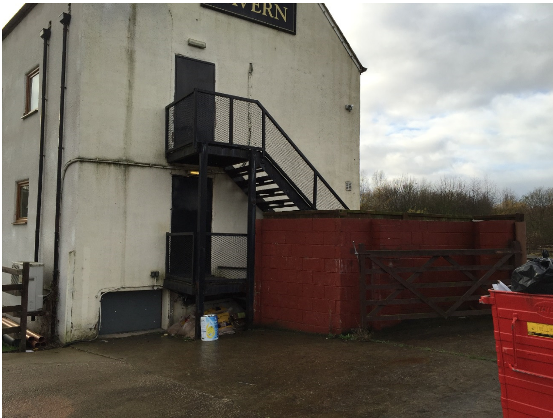
View to the side (north) elevation showing existing steel escape staircase & boundary treatment
