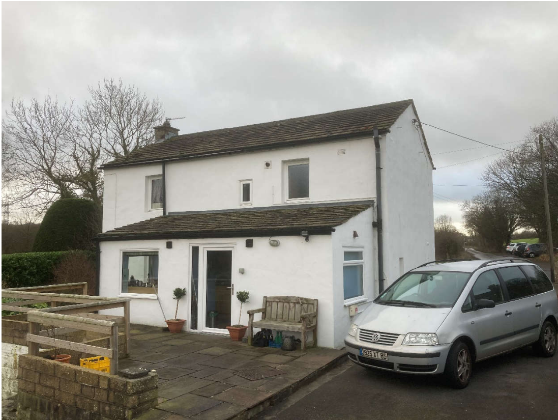
05. Rear, north east elevation and north west gable looking from rear.
