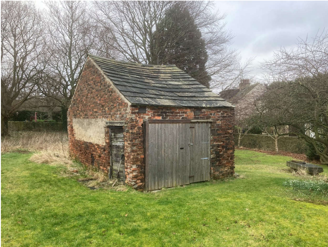
09. Brick garage with slate roof – front (west) and left gable (north).
