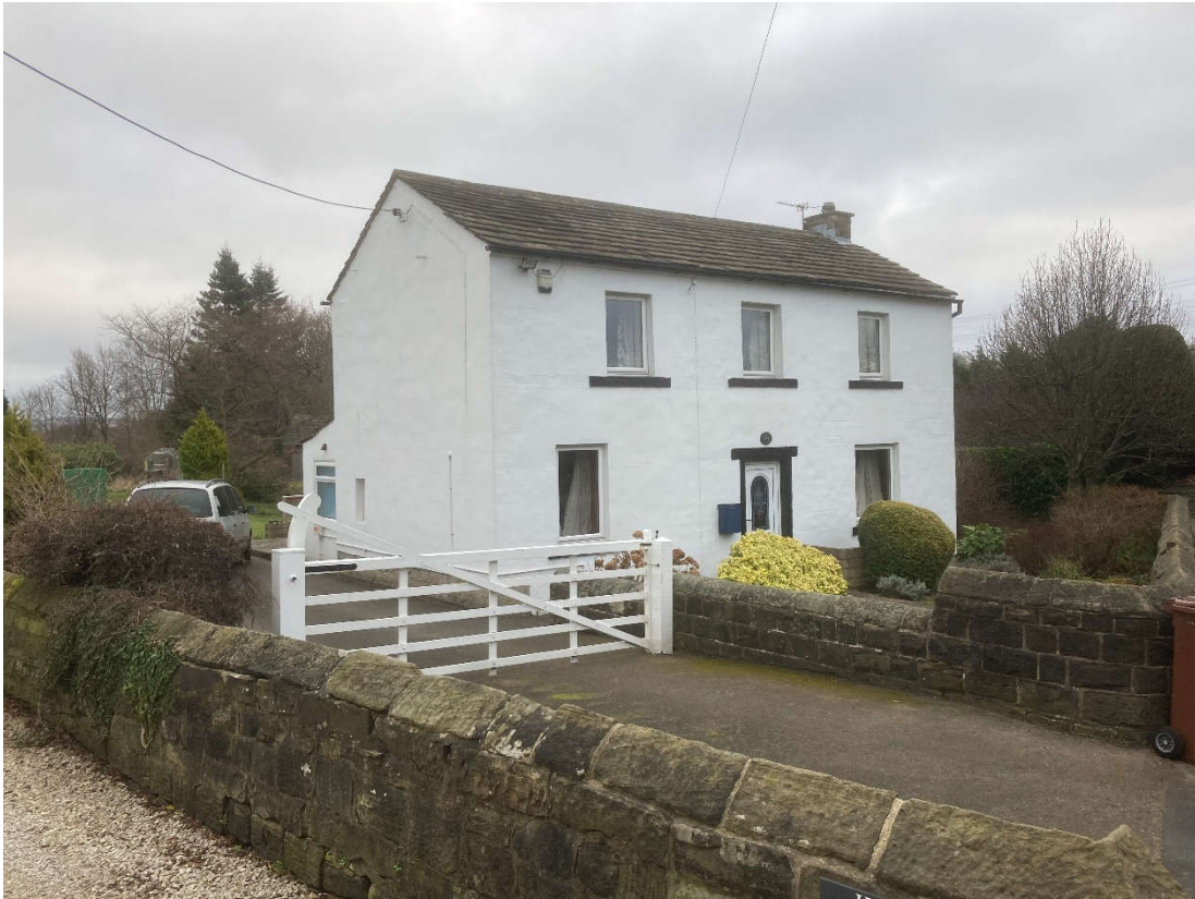
03. Access drive and gate, north west gable elevation.
