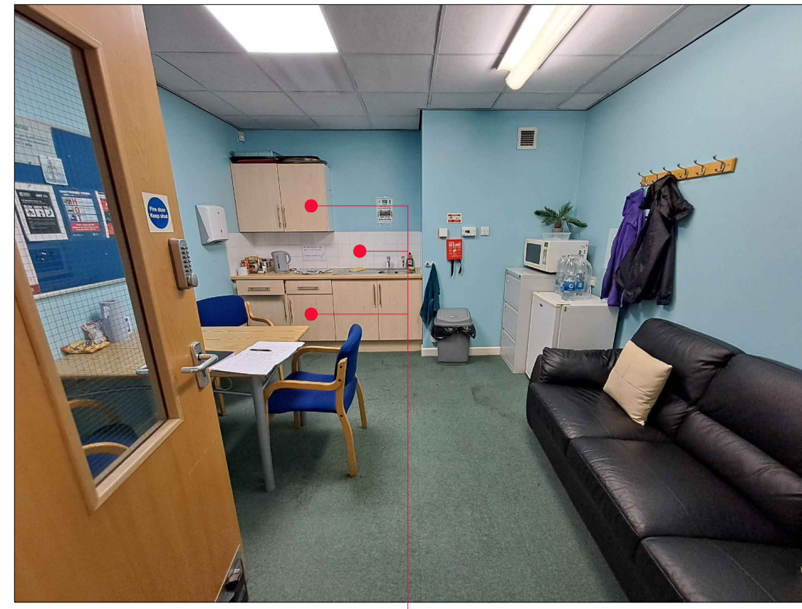
Photo 13 Staff Room / Kitchenette - Remove existing kitchen units including wall cupboards, worktop, base unit cupboards, inset sink and drainer. Remove ceramic tile splashback and make good to disturbed plaster.
