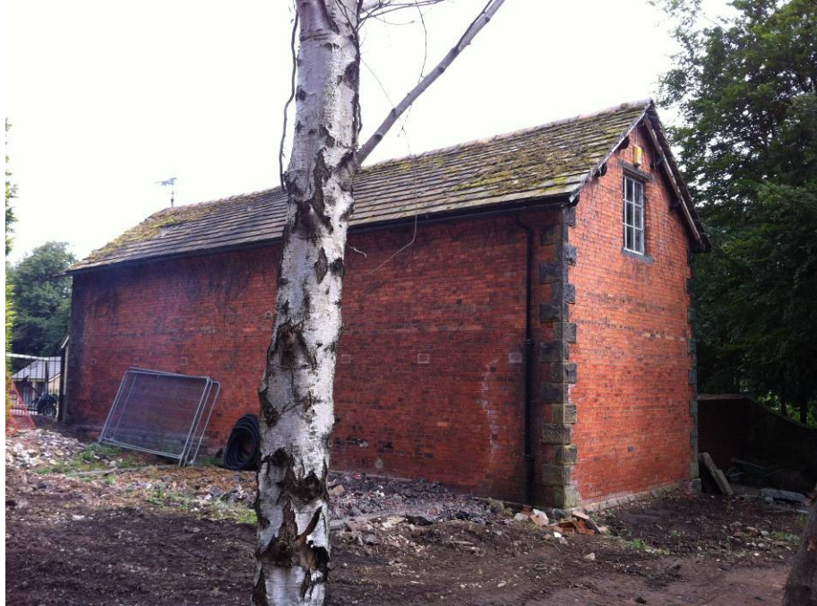
Fig 3. South gable and West Elevation
