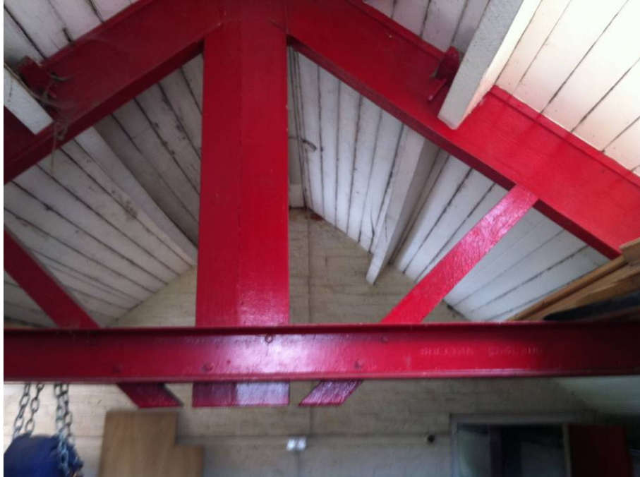
Fig 5. Truss 1 showing steel beam replacing bottom tie of timber truss.
