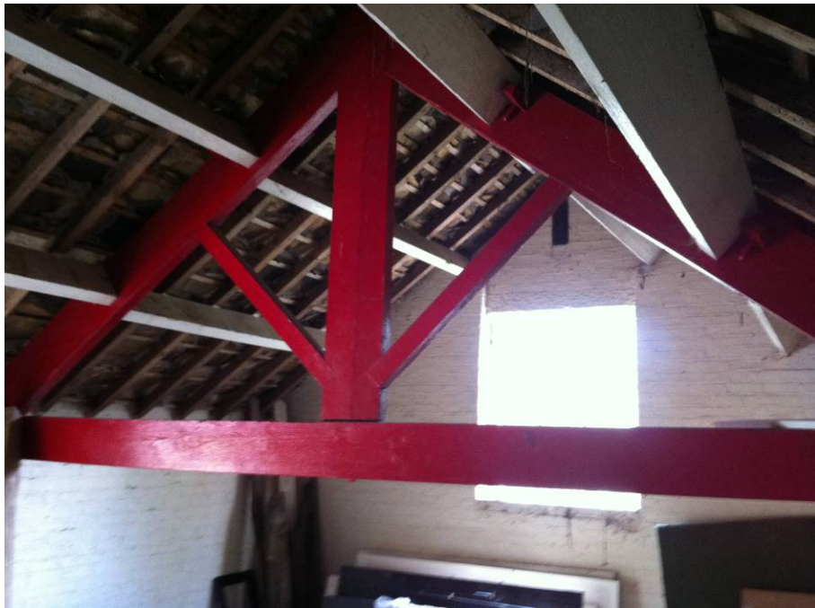
Fig 6. Truss 2 and purlins in original condition.
