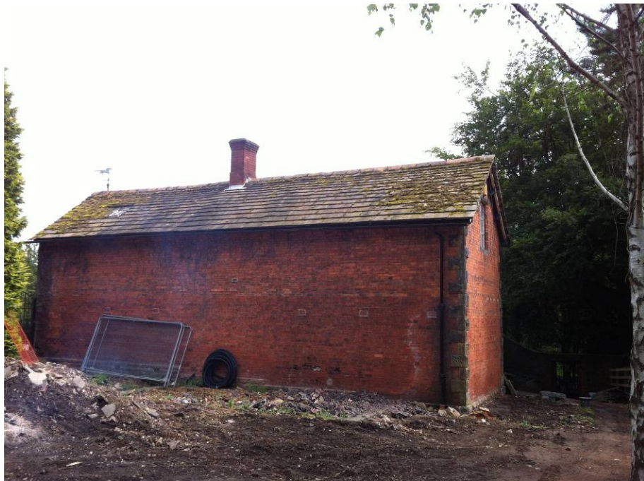
Fig 4. West Elevation showing chimney stack and rooflights.
