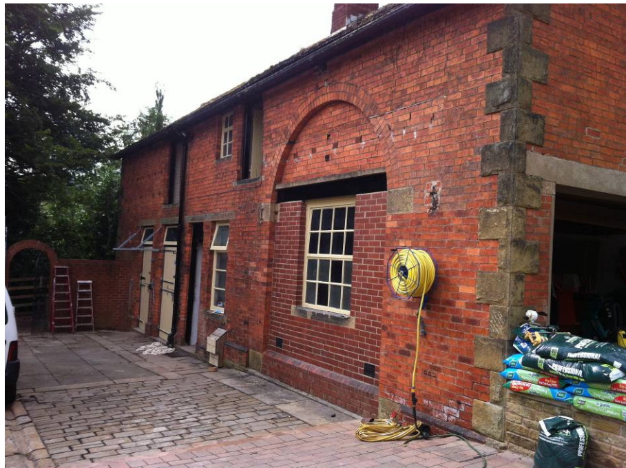
Fig 2. East Elevation of Barn showing arched opening currently built up.
