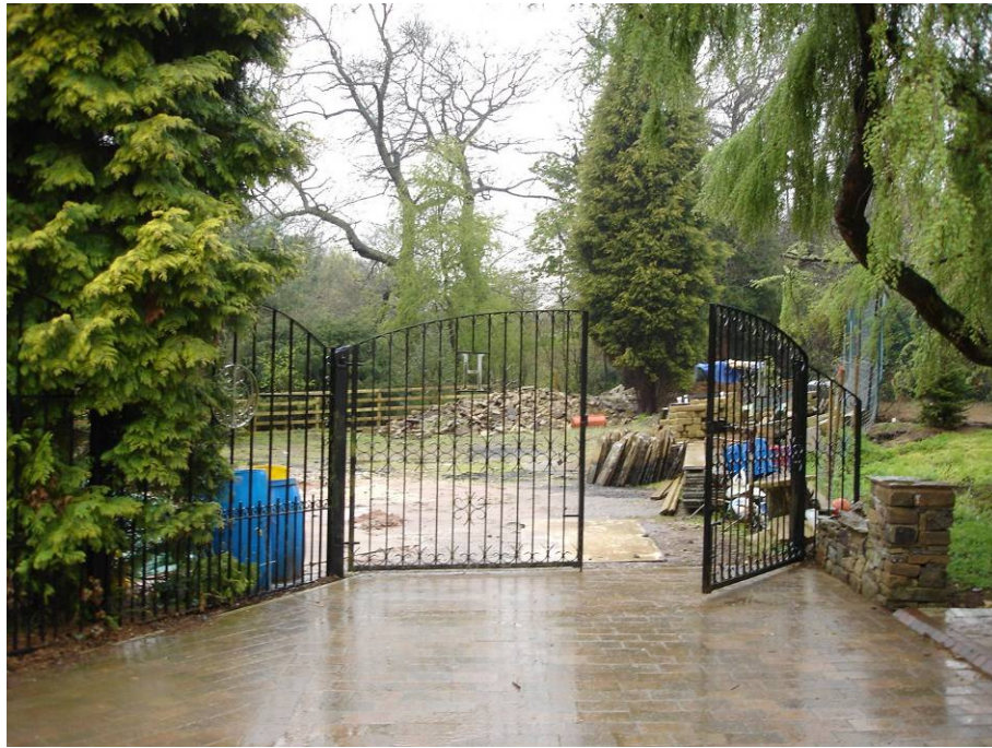
Fig 7. Existing access gates to land at rear (west) of Barn.
