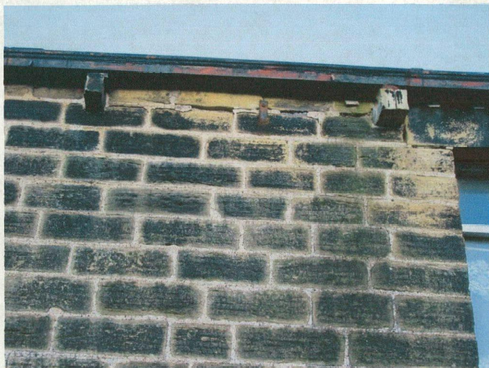
Photo 1 – Extensive weathering of slats to No's 3 on left and 321 in the centre. Bricked up first floor window above old Post Office frontage.
