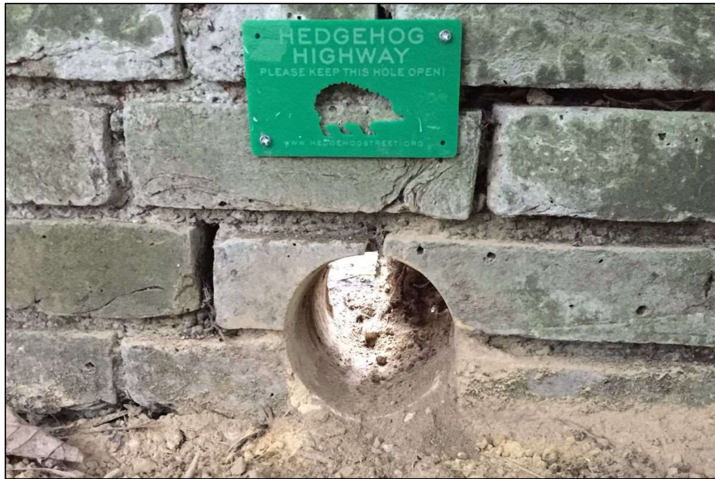
Plate 6. Hedgehog hole in a boundary wall with signage to identify its purpose. 7
