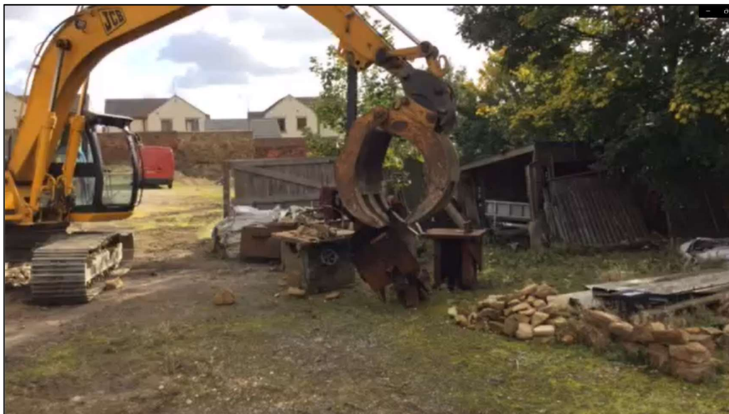
Plate 1. A photo of the site taken during the demolition of the barn in 2019 showing ephemeral vegetation on hardcore across most of the site
