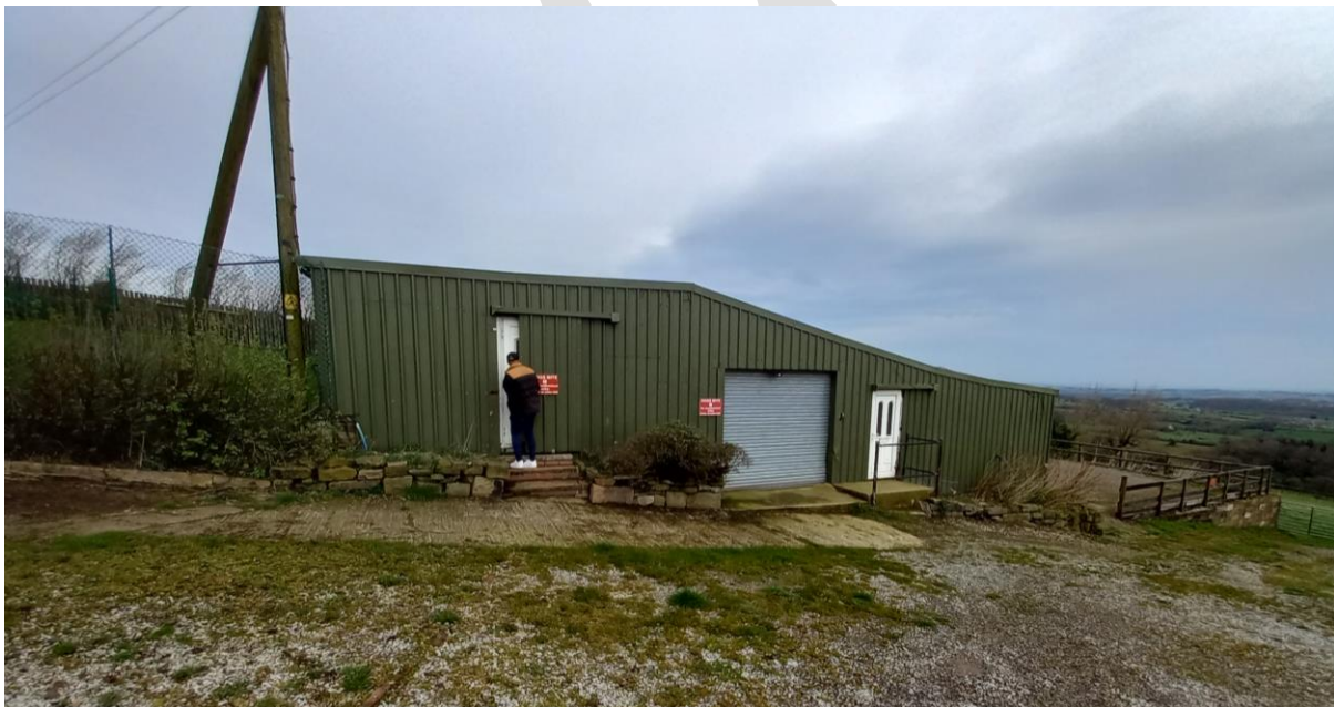
View of former kennel
