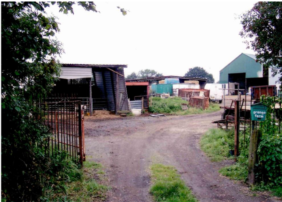
VIEW TO FARM BUILDINGS FROM ENTRANCE
