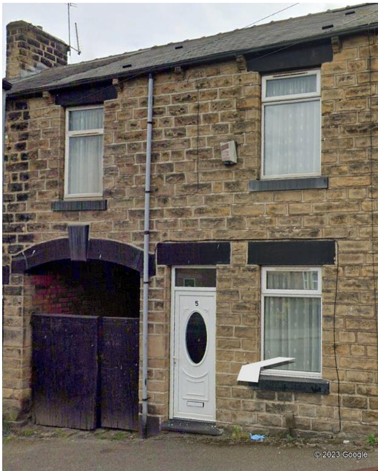
5 Tune Street - Front elevation image
