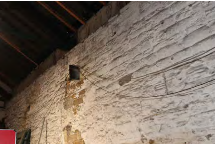
Building 20, thick impermeable paint to stonework
