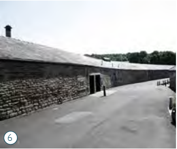
6 Retail and Storage Former Workshop Grade II* Listed
