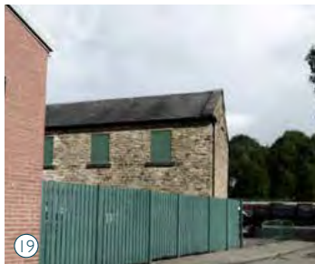
19 Store Former Locomotive Shed Grade II* Listed
