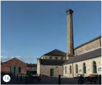
16 WCs Former Boiler House Grade II* Listed
