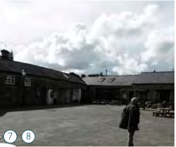
7 8 Retail and Storage Former Workshop Grade II* Listed
