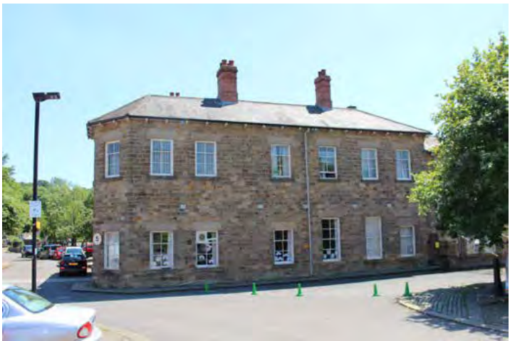
Building 13, northwest elevation
