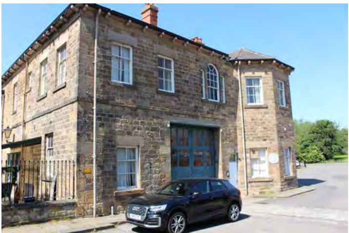
Building 13, northeast elevation
