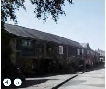
4 5 Retail and Storage Former Workshop Grade II* Listed
