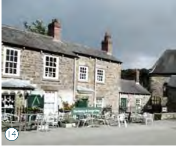
14 Cafe Former Cottages Grade II* Listed
