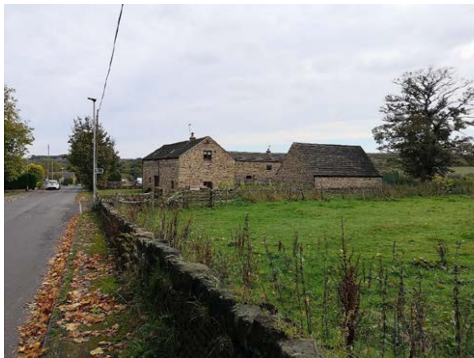
Listed barn, looking east along Hay Green Lane
