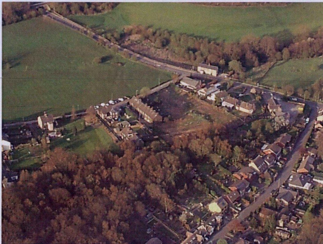
Figure 2.5 Aerial view demonstrating the infill characteristics of the site
