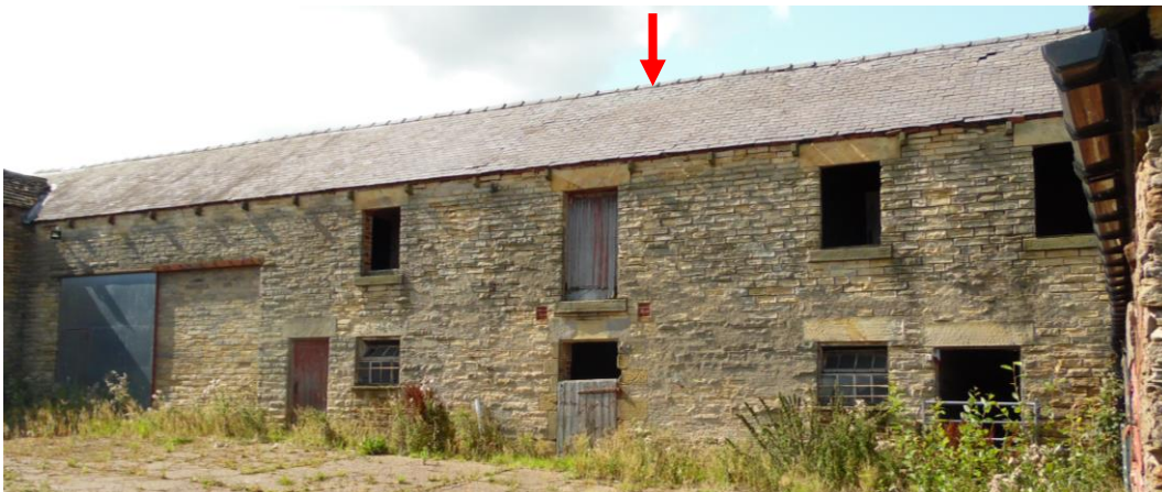
Figure 8 Approximate location of roost in ridge of barn (building 6).
