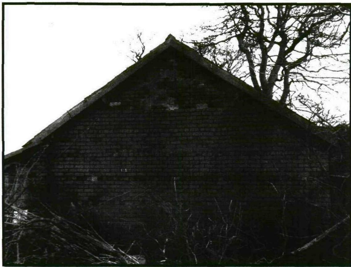
Photograph 40 – View of West Elevation
