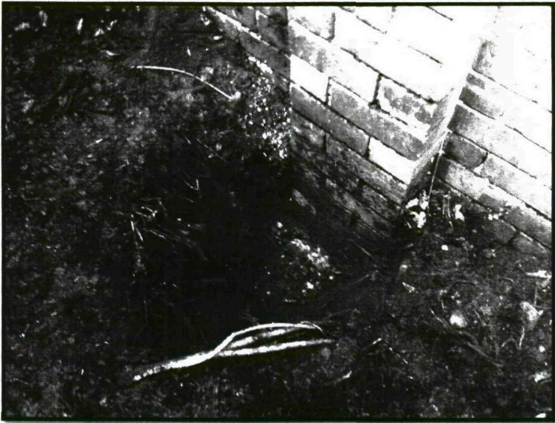
Photograph 43 – View of trial pit on South Elevation
