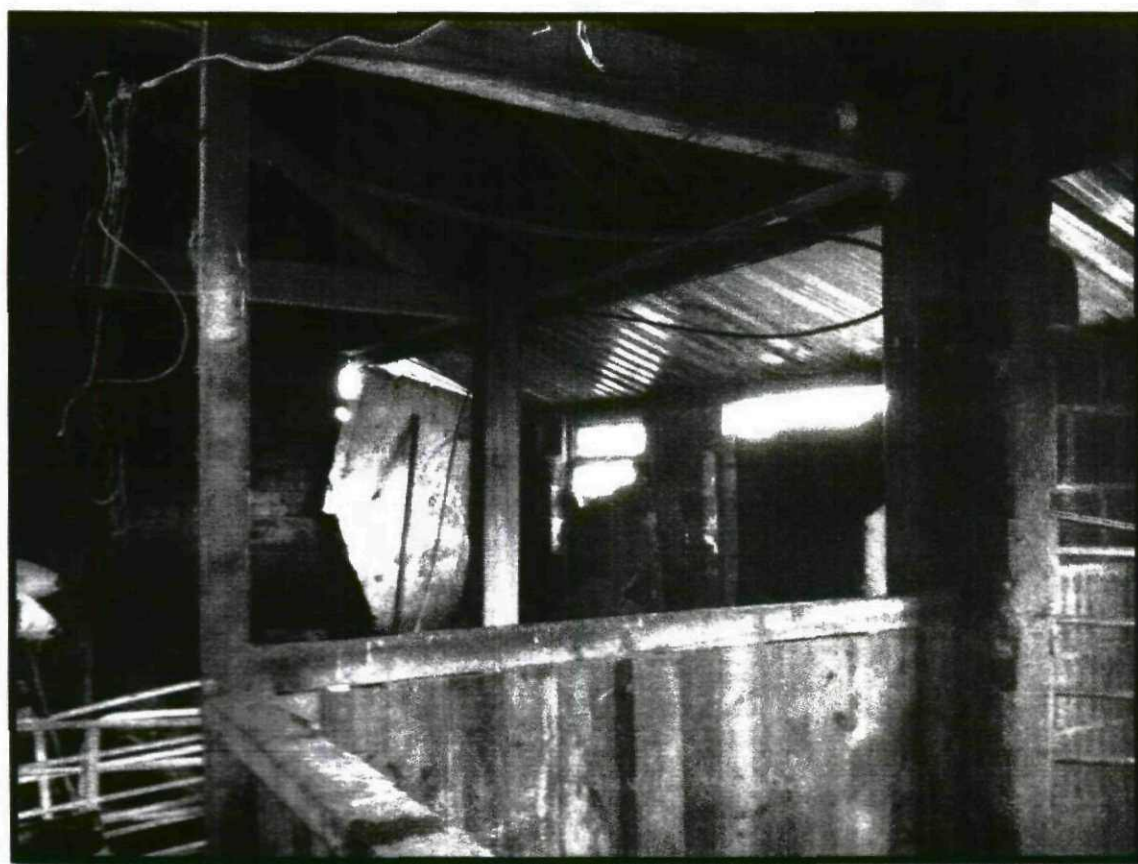
Photograph 48 – Showing timber columns and beams supporting North edge of roof
