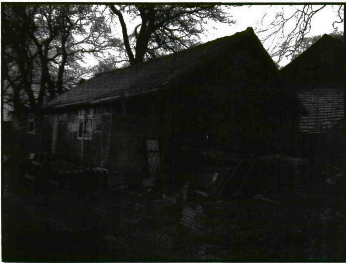
Photograph 44 – View of North Elevation
