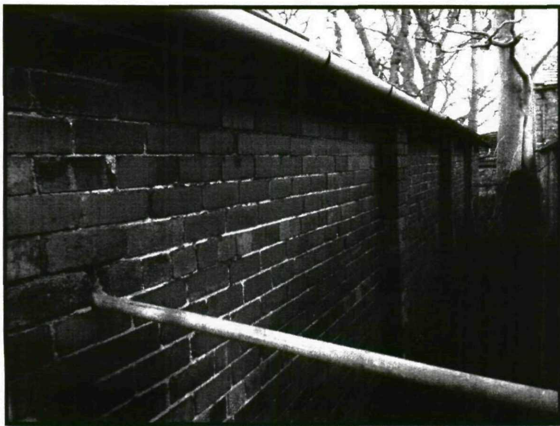
Photograph 42 – View of South Elevation
