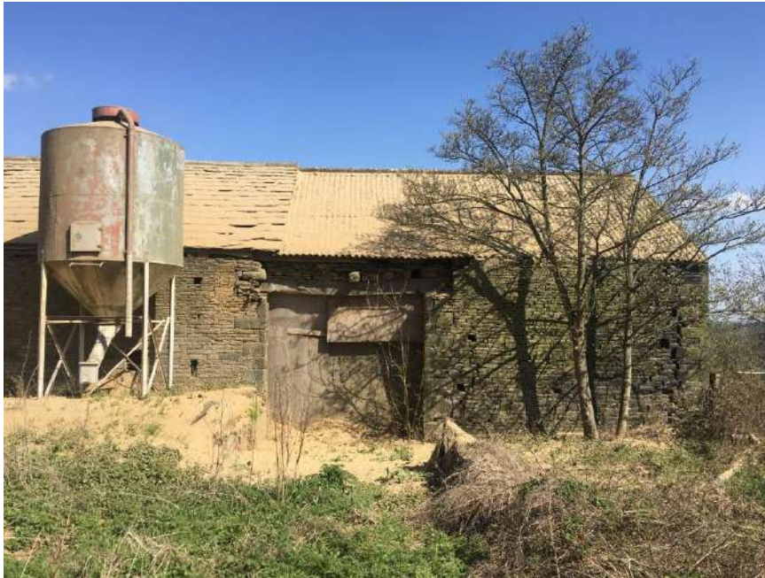
Extent of profiled sheeting to Unit 3
