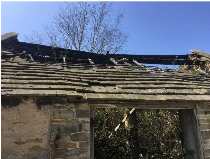
Front roof slope to Unit 1
