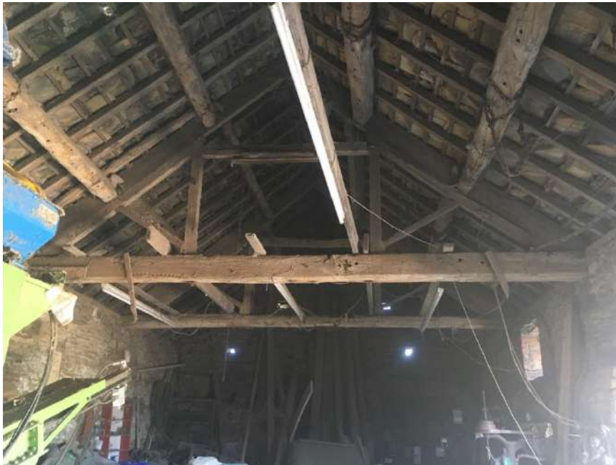
Roof trusses within Unit 3.
