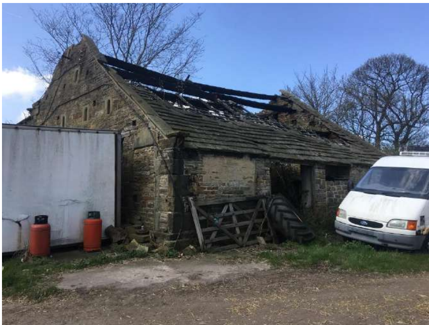
Unit 1 view from south east
