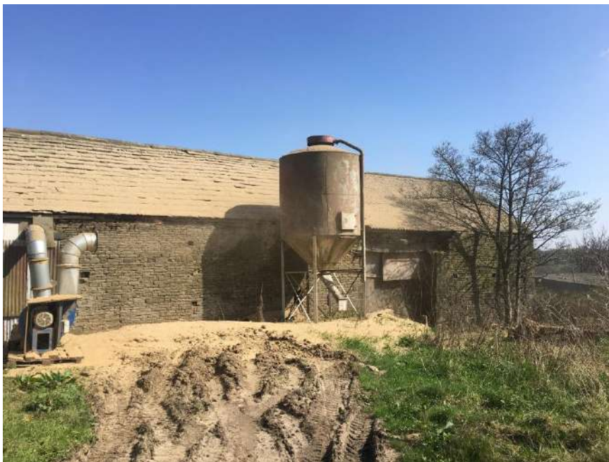
Rear photo of Unit 3. Viewed from West
