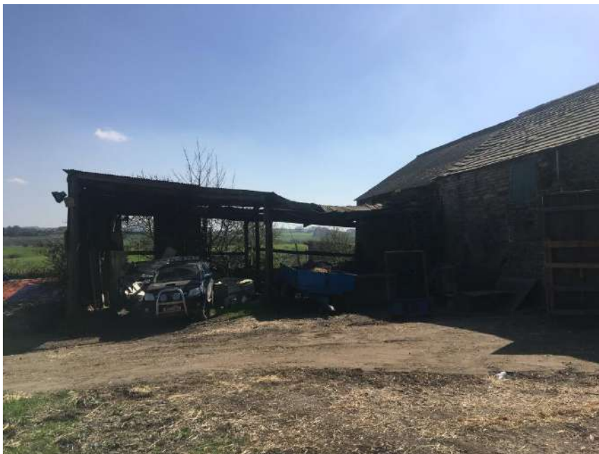
Perpendicular pole building to East of Unit 3 (to be removed)
