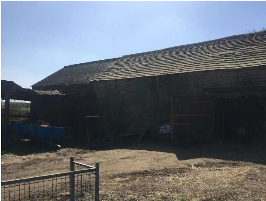
Unit 3 Viewed from North East
