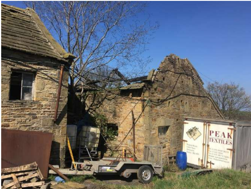
Gable of Unit 1 & front of Unit 2
