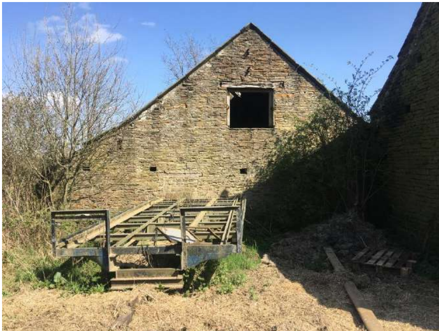
Unit 2 gable viewed from West
