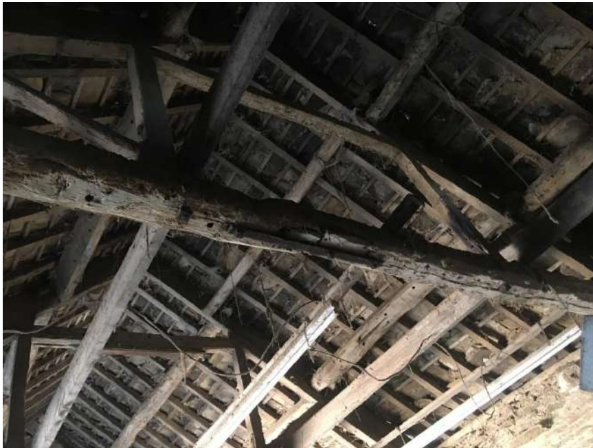
1 st truss within Unit 3.
