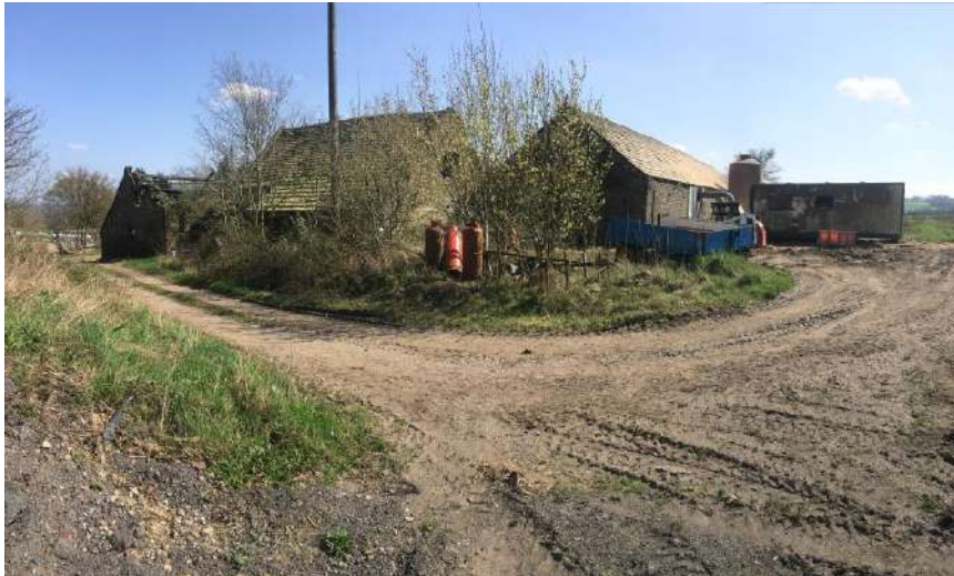
Panoramic view of Unit 1, 2 & 3
