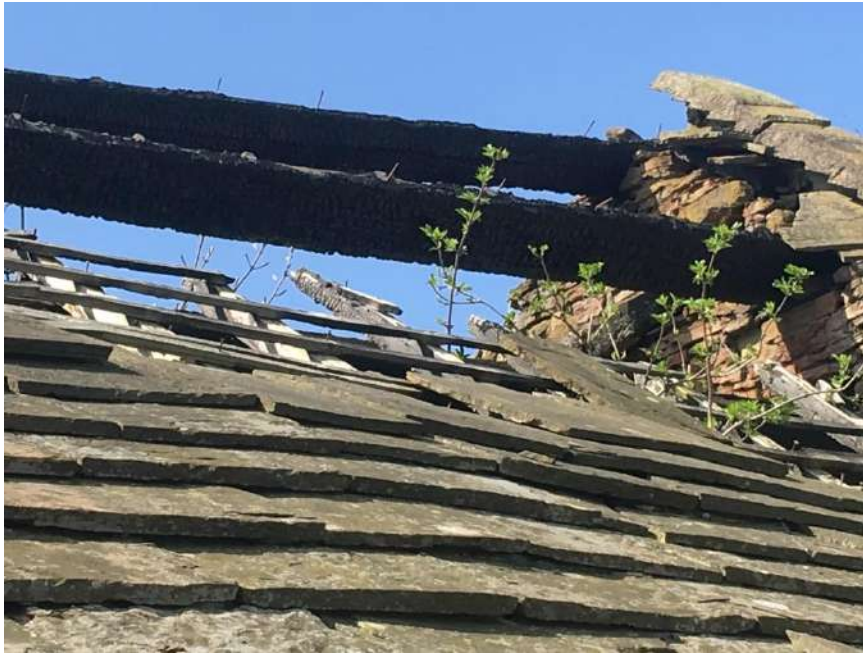
Charred front roof slope timbers to Unit 1
