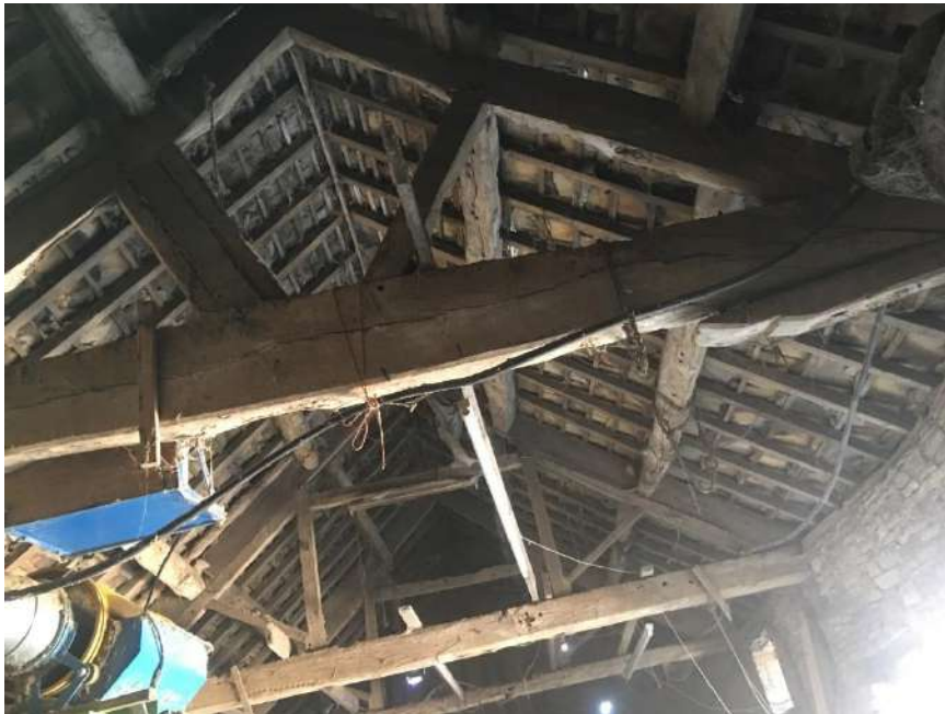
Roof trusses within Unit 3.
