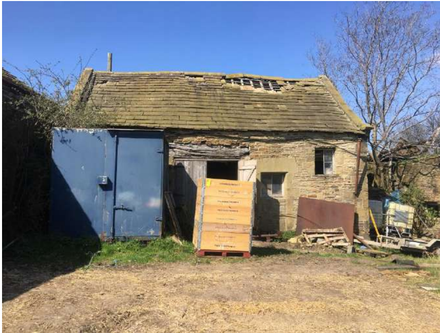
Unit 2 Front. Viewed from South
