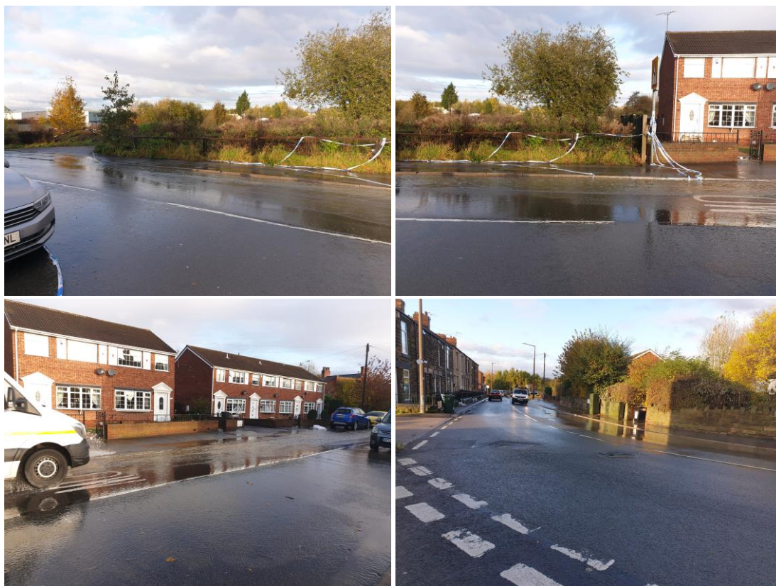
Figure 1: Flooding on Station Road
