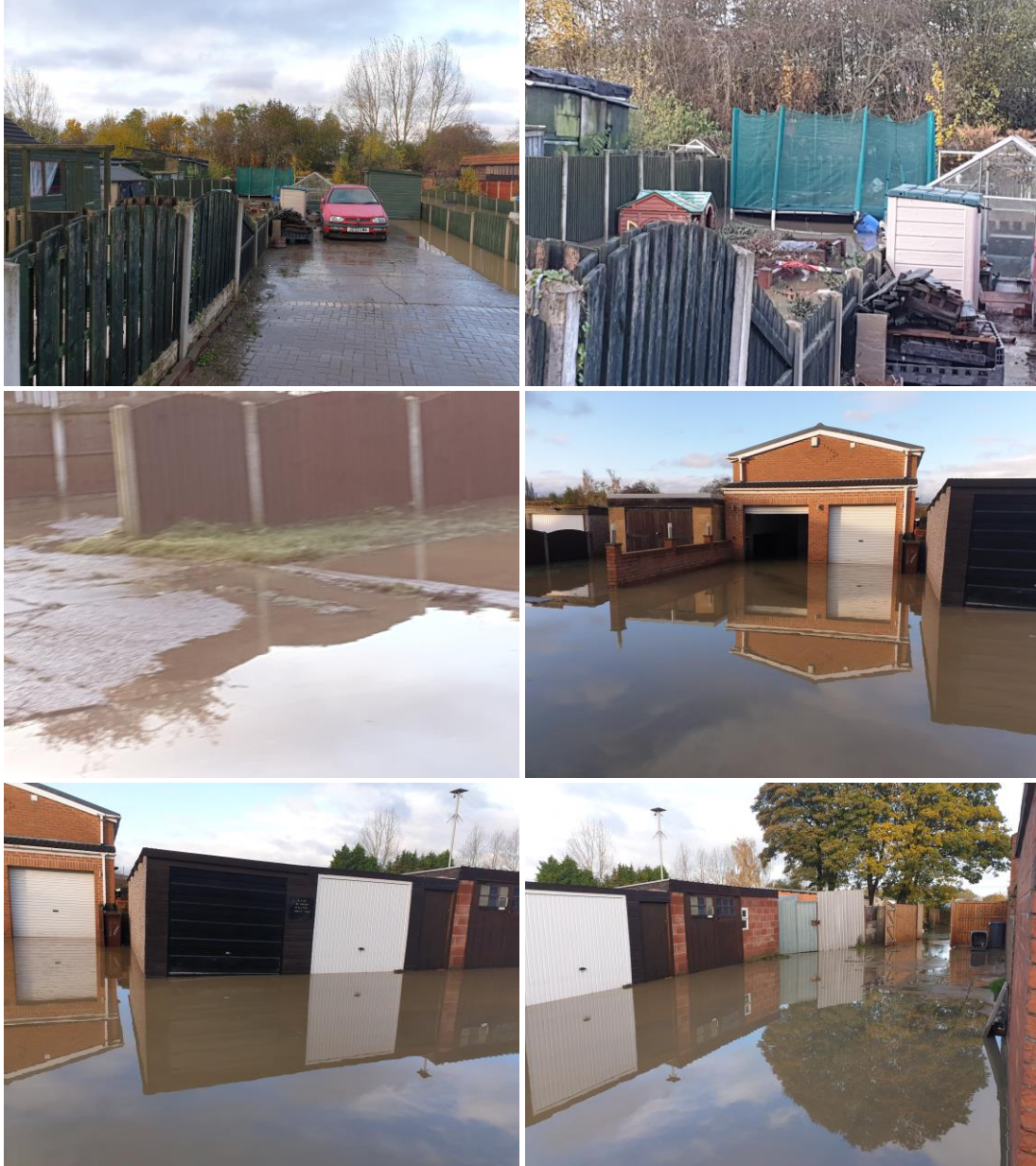
Figure 3: Flooding to properties on Stonyford Road
