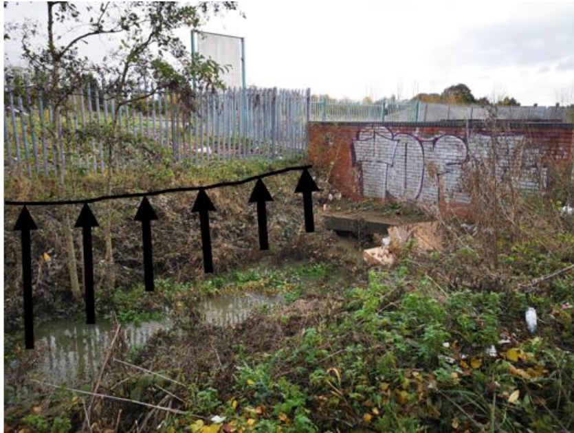
Figure 10: Bulling Dyke wrack mark upstream of Valley Road access bridge
