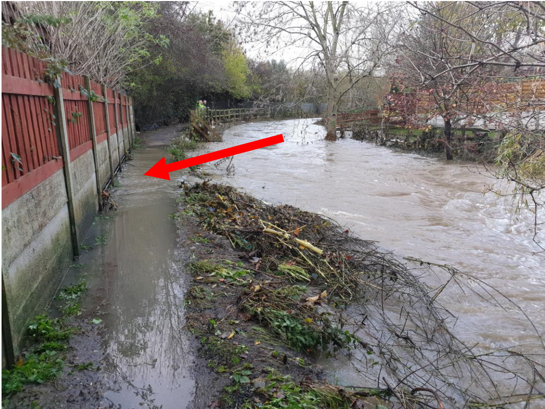
Figure 4: Right bank flooding on the River Dove upstream of Stonyford Road
