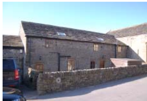
The conversion &amp; Courtyard
