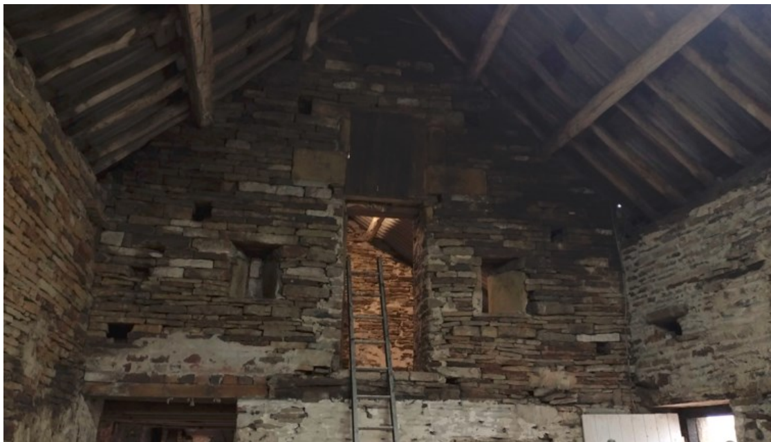
Within bay 4 looking north towards enclosed gable wall
