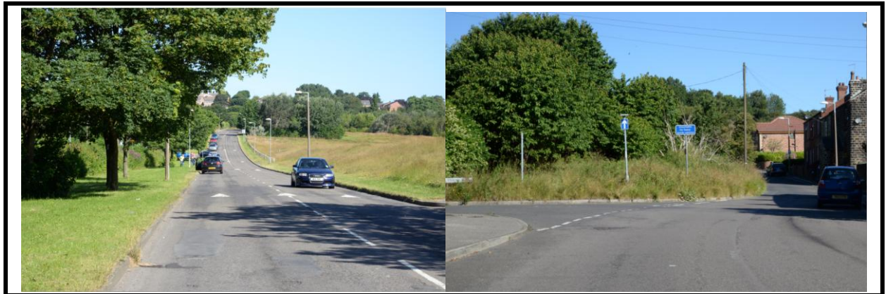
Littleworth Lane northerly towards the one way section
