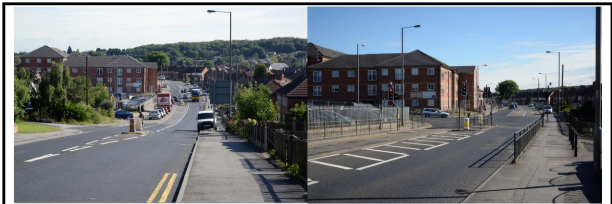
Pontefract Road easterly towards the signalised crossing with pedestrian facilities.
