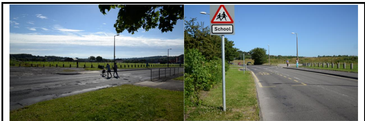
Crossing location Littleworth Lane
