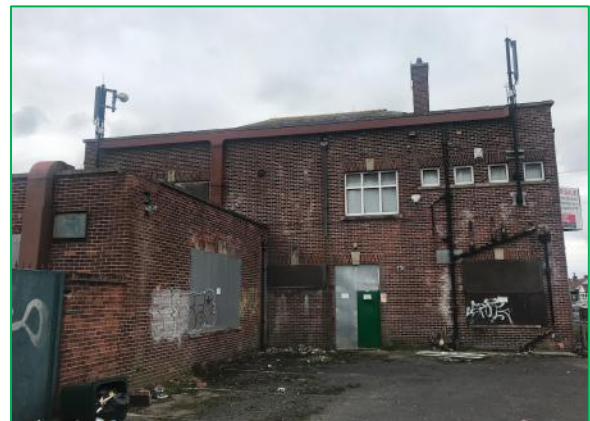
The east elevation of the building
