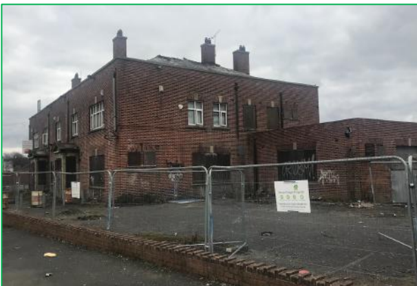
The north and west elevation of the building
