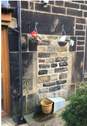
Infilled Existing Front Door
