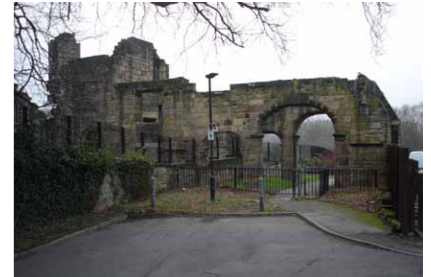
Photo 2: looking south to Priory and footpath link
