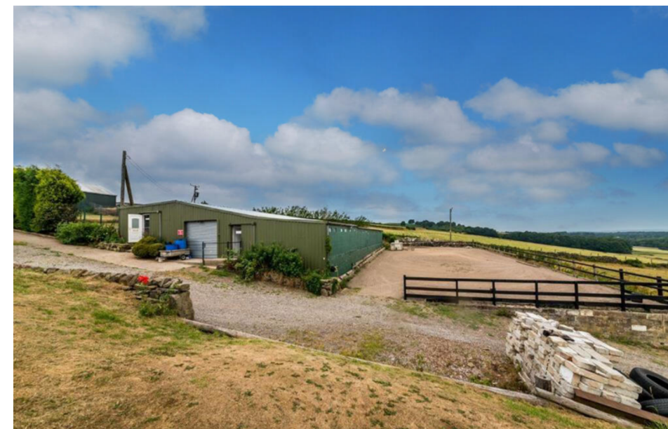
Southeast elevation view of the building noting the sloping ground.
